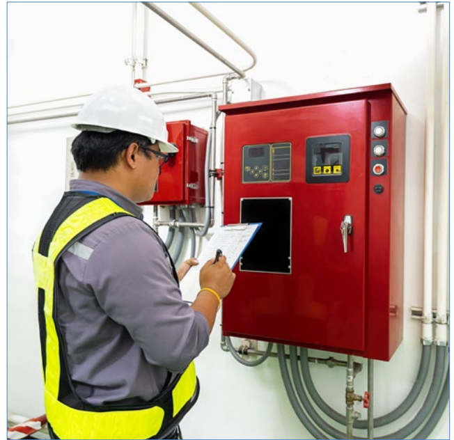
Figure 5. Our comprehensive fire safety inspections ensure that fire safety systems and equipment are up to code.
