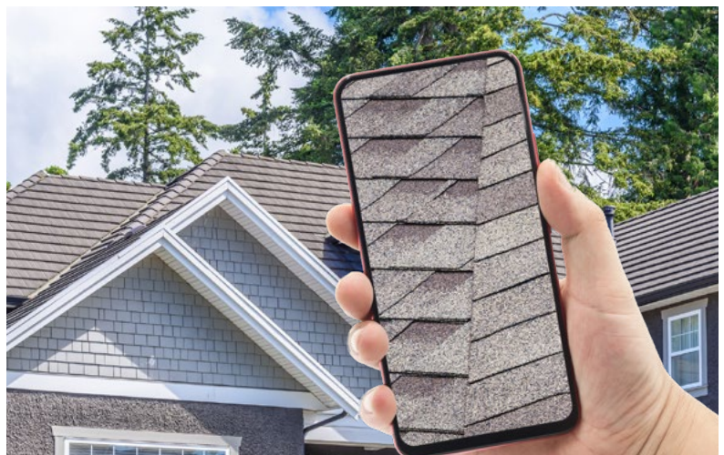
Figure 4. Climbing up on a roof for an inspection is a risky and time-consuming job. RVIs are ideal for performing roofing inspections safely.
