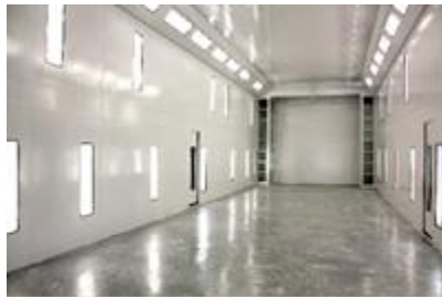
CWD's on-site truck/container paint facility
