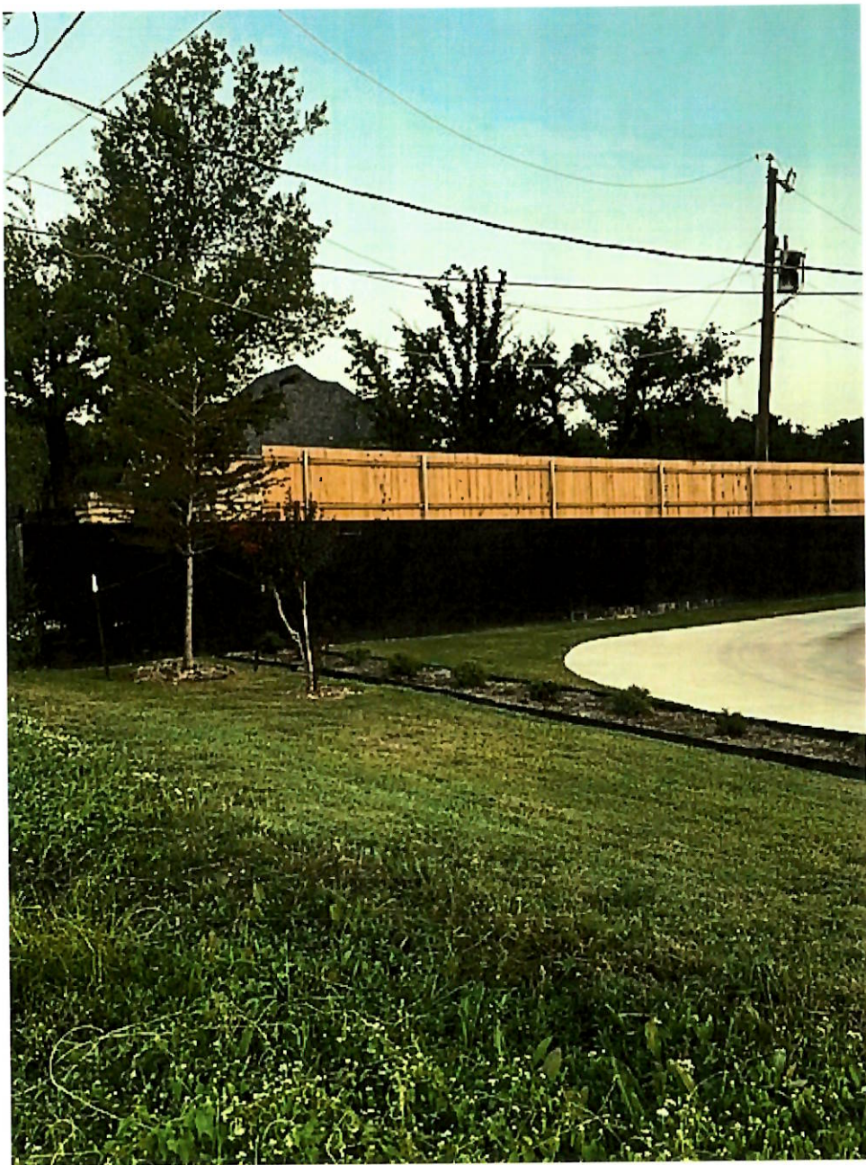
VIEW FROM COMMERCIAL PROPERTY AFTER FENCE INSTALLATION
