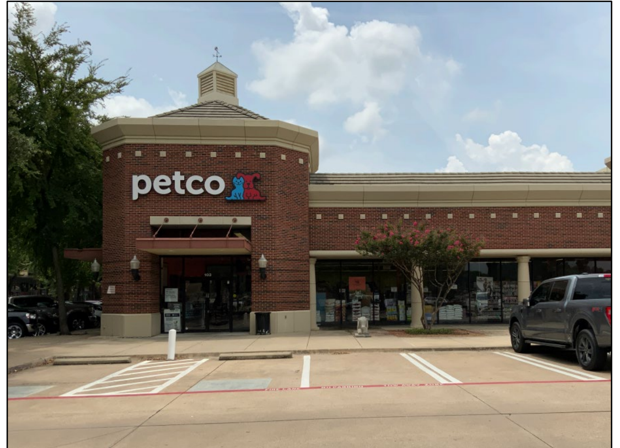
Proposed location at 1006 Keller Pkwy.
