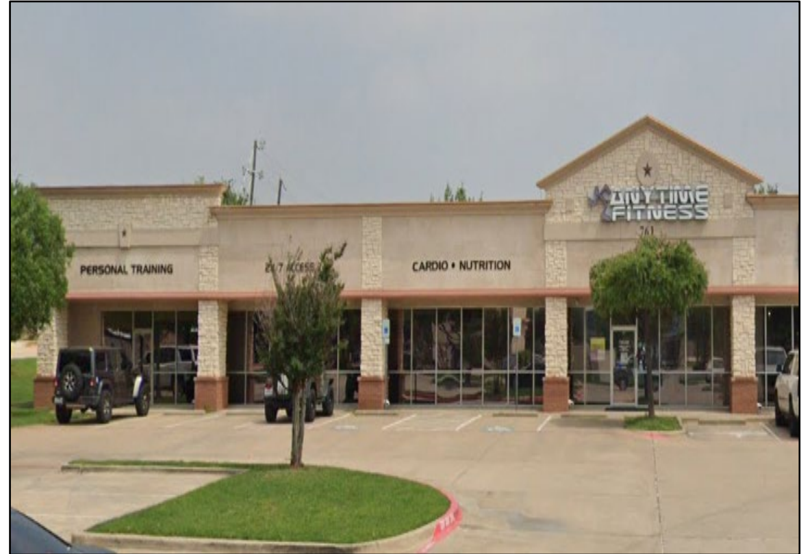
Proposed lease space at 761 Keller Pkwy., Unit 104
