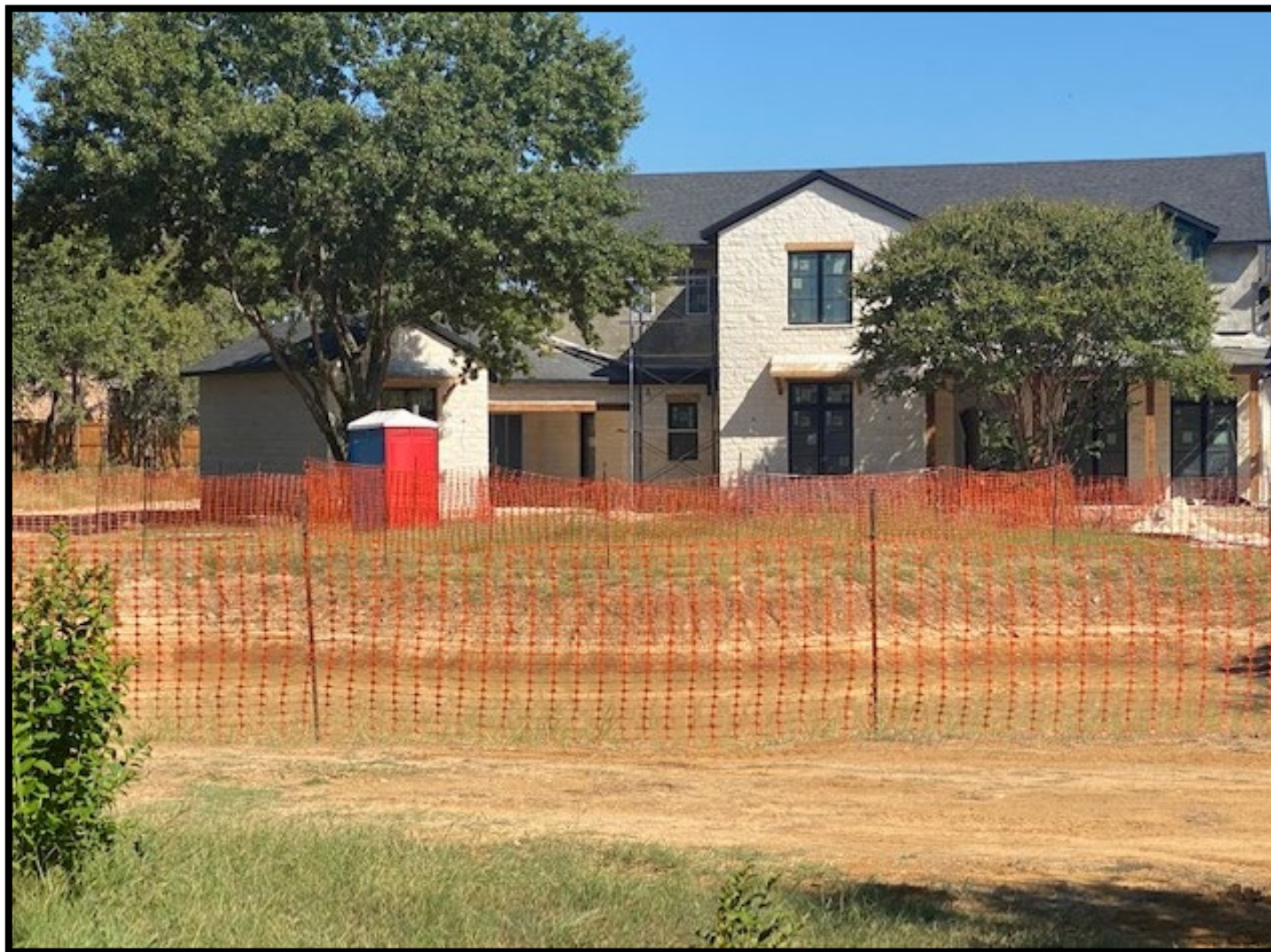
New home under construction
