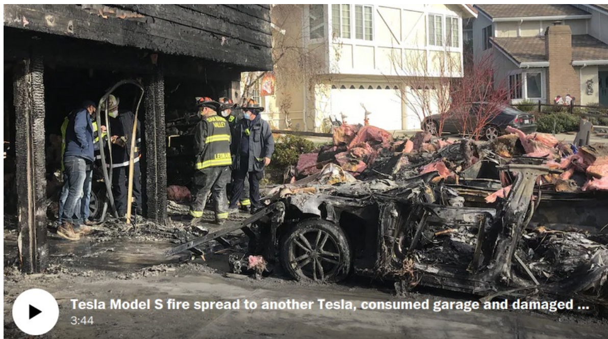
Figure 25: EV fire destroys home garage
