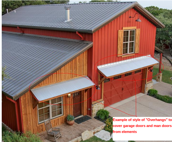
Photo 1 - Example of "overhang" to protect garage and man doors from elements.
