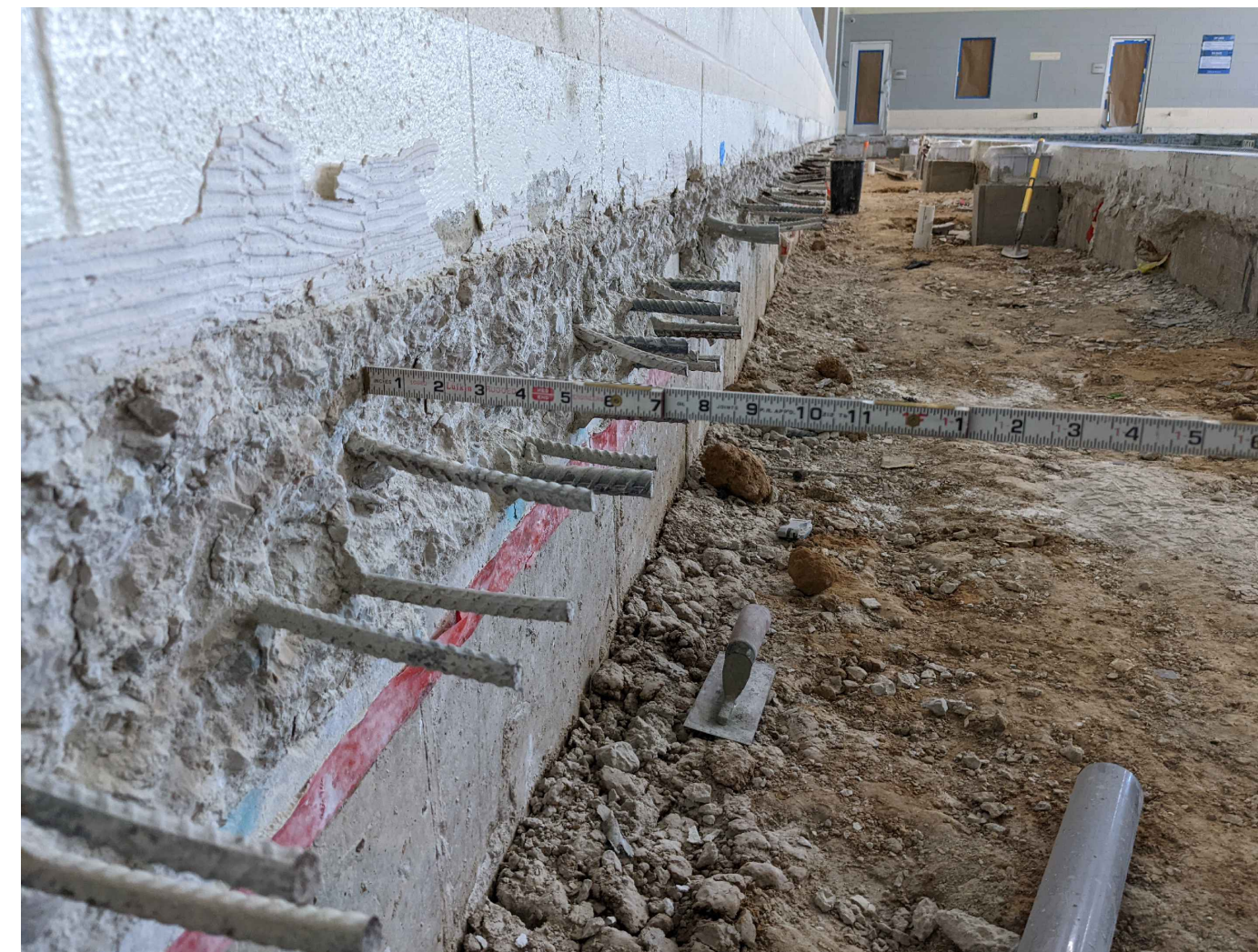
PHOTO 3 - CLOSEUP OF BAR STUBS AT SOUTH WALL
