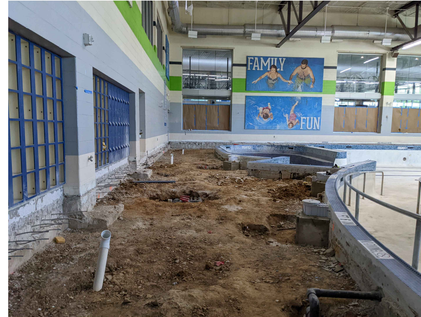
PHOTO 1 - LOOKING SOUTH ALONG EAST WALL
