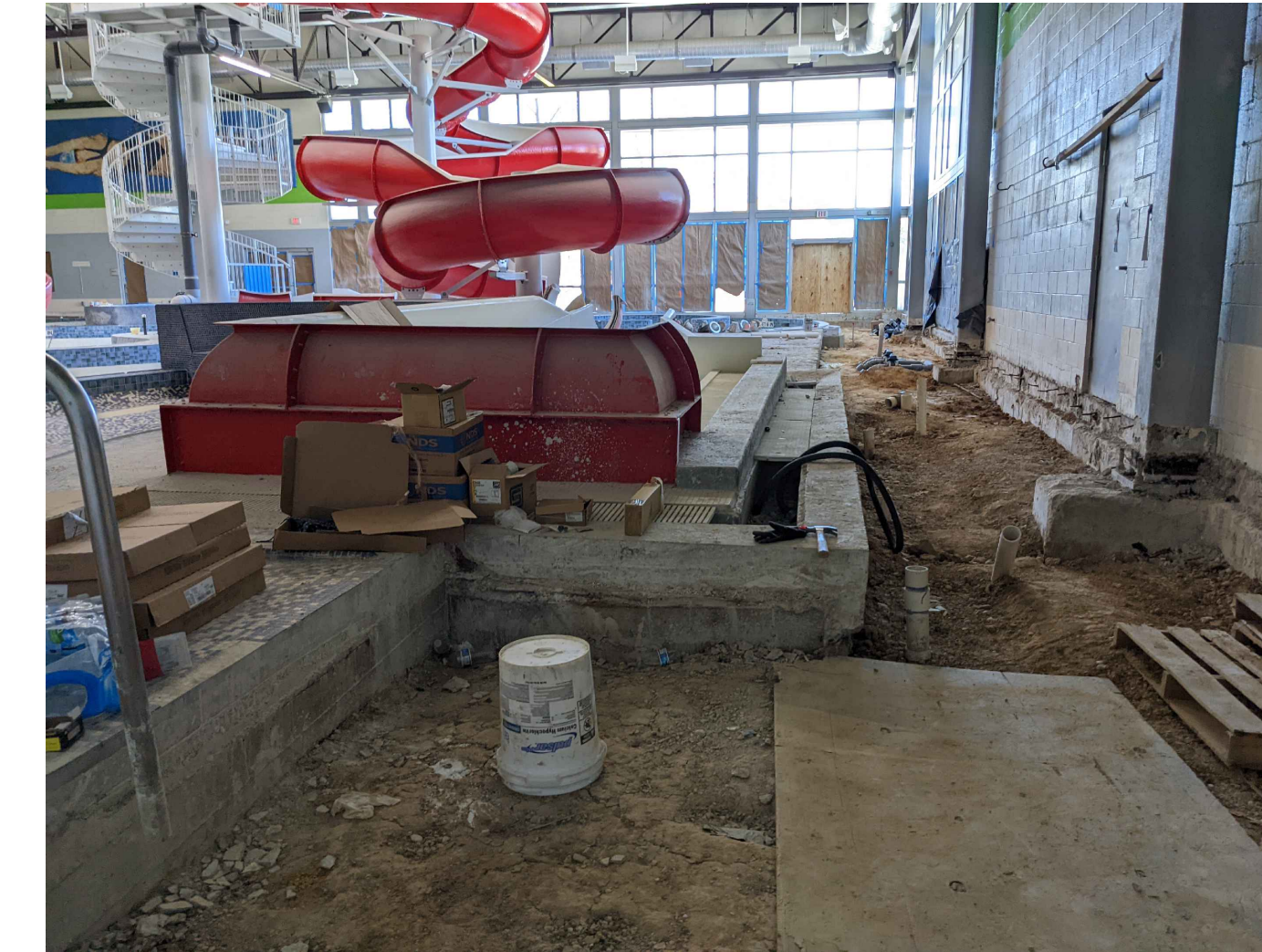
PHOTO 2 - LOOKING WEST ALONG NORTH WALL
