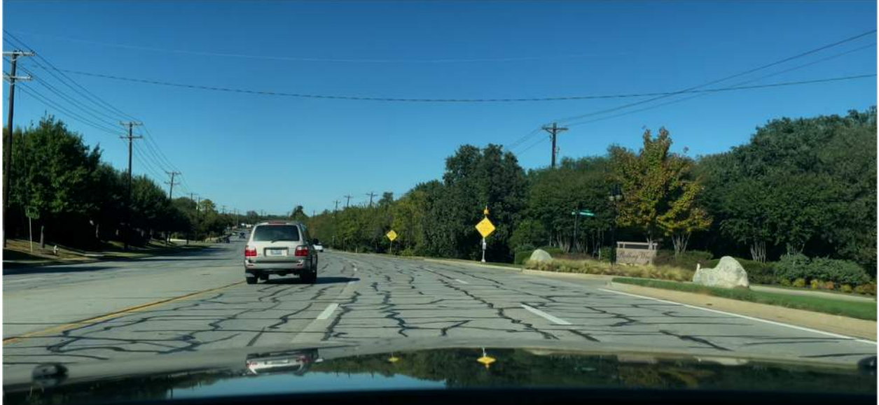
Northbound Davis Blvd (FM 1938) (425' south of Street A)
