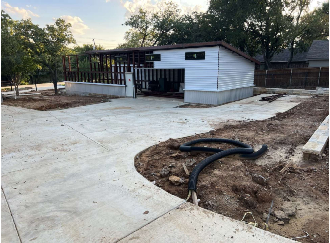
2025 current status of structure
