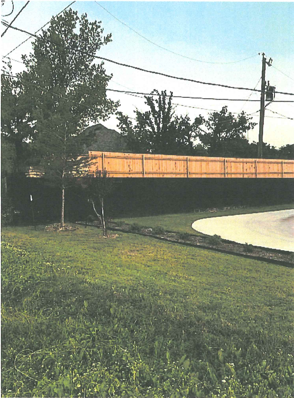
VIEW FROM COMMERCIAL PROPERTY AFTER FENCE INSTALLATION
