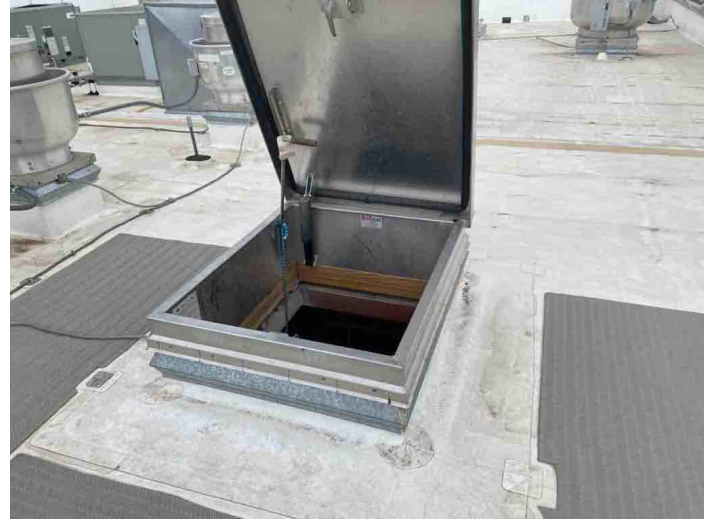
Group: 1.6 - Category: Roof Access
