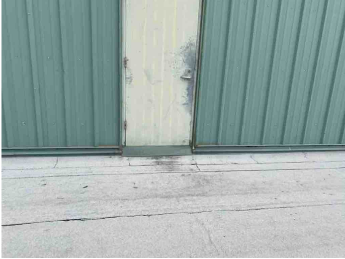
Group: 1.5 - Category: Roof Access
