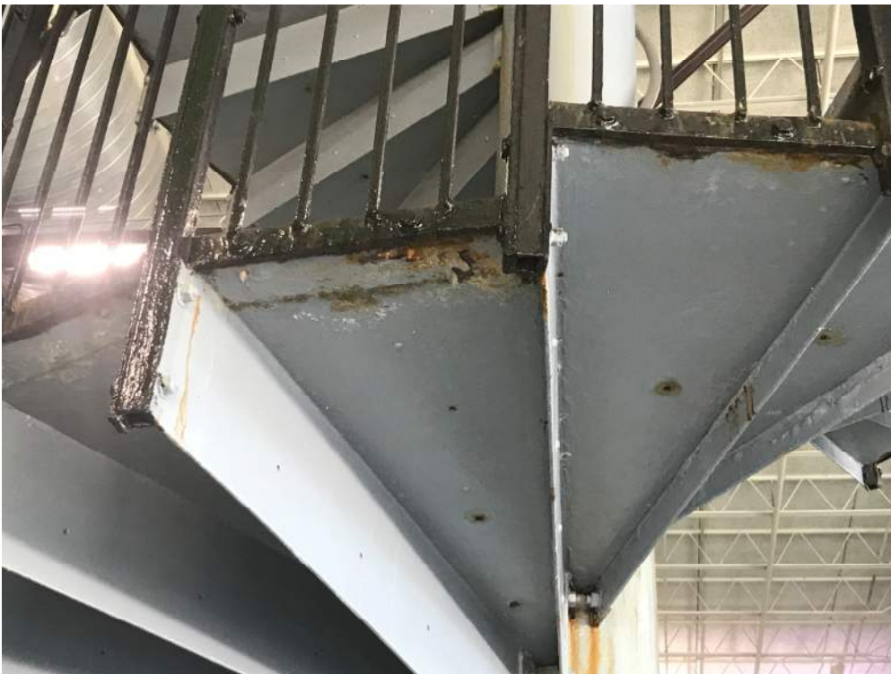
Example of Rust on Spiral Stairs and Railing
