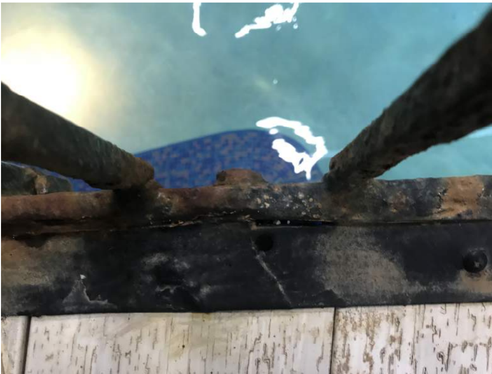
Example of High Corrosion on Railing at Slide Platform
