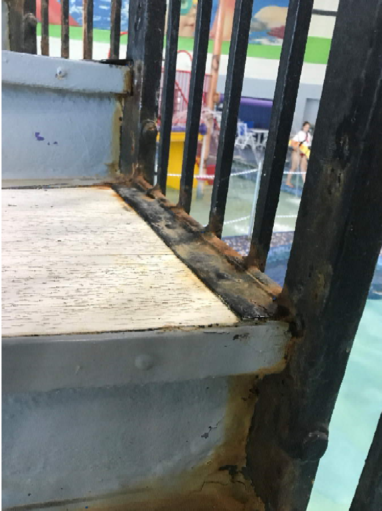
Example of Rust on Stairs and Railing
