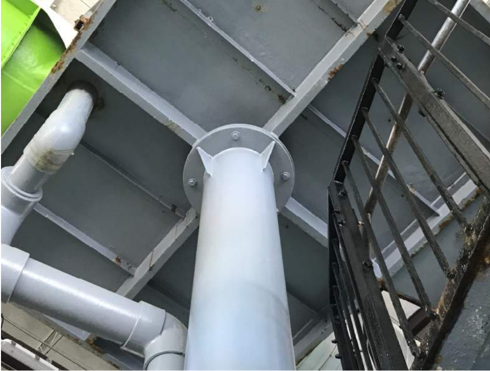
Example of Tower Rust and Chipped Paint
