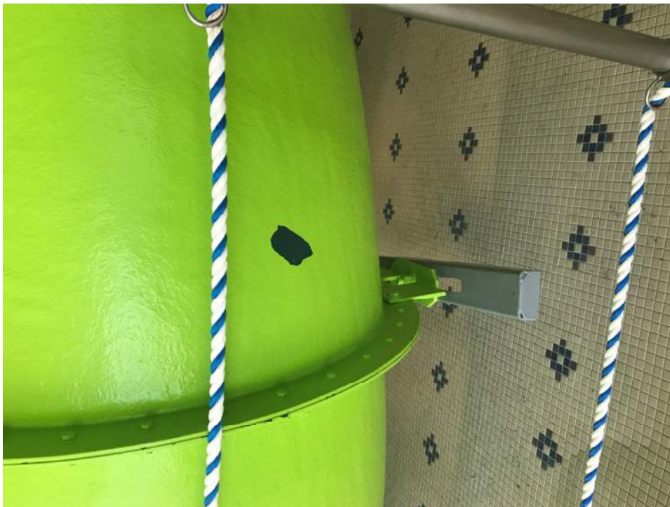
Example of Chipped Gel Coat on Slide
