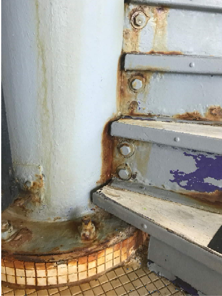
Example of Spiral Stair Connection Rust
