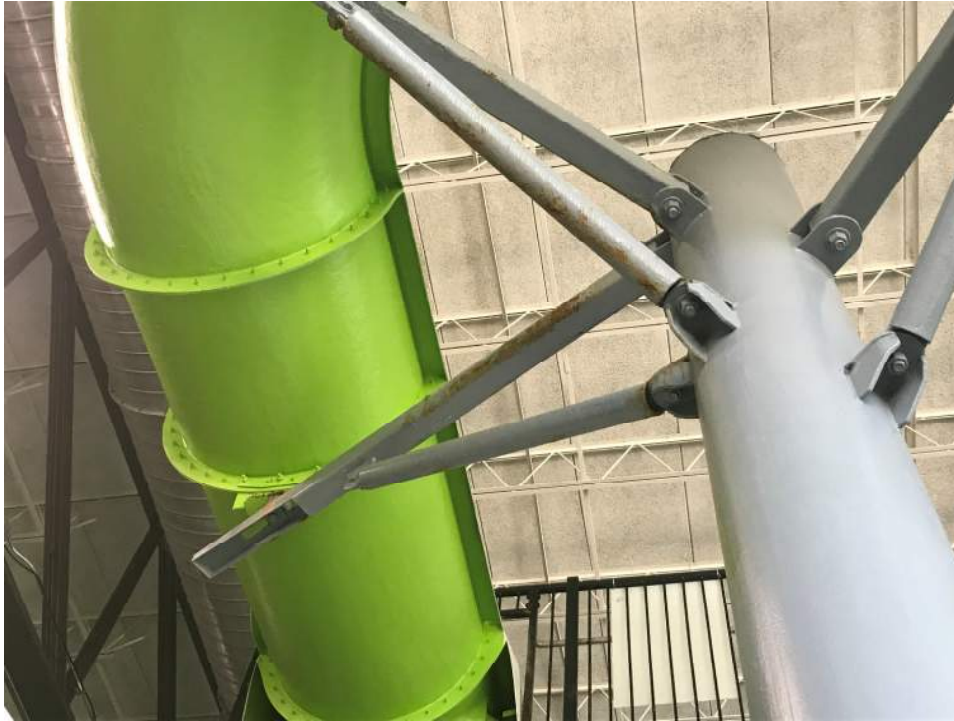
Example of Rust on Slide Support Arms
