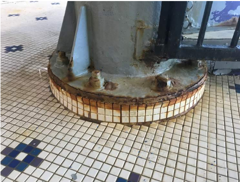
Example of Bolt Rust on Spiral Stair Column Anchor Bolts
